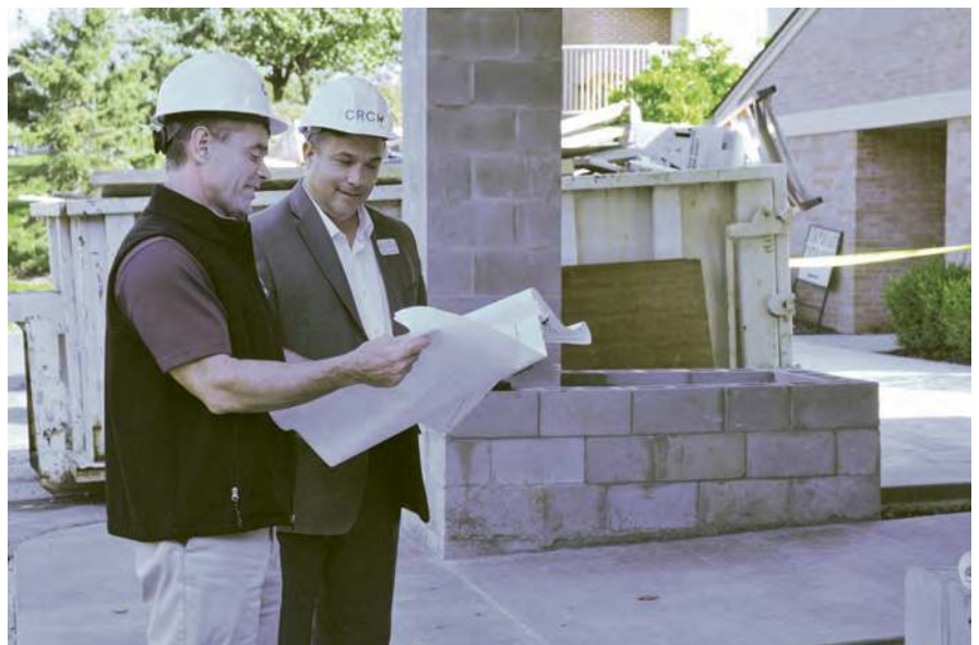
Dan Rhodes, president of the construction company CRC, Inc., and Home executive director David Chappell confer about renovation progress at the building entrance.
