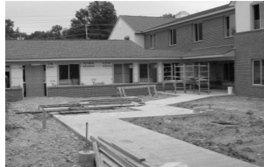
Willow Brook Christian Home construction progress as of September 3, 2004.
